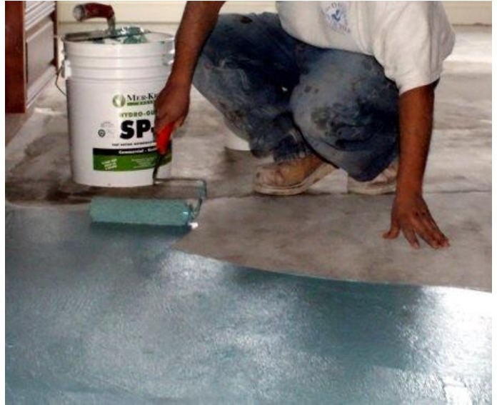
Hydro Guard SP-1 application for Crack Isolation prior to tile installation
