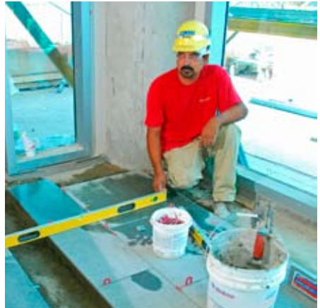
Work moves forward on the main lobby floor.
