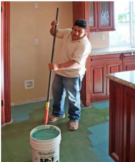
*Hydro Guard SP 1 ensures waterproof, crack-resistant surfaces in high traffic areas.*
