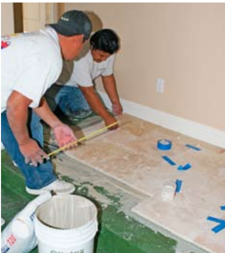
Installers take the full measure for quality workmanship.
