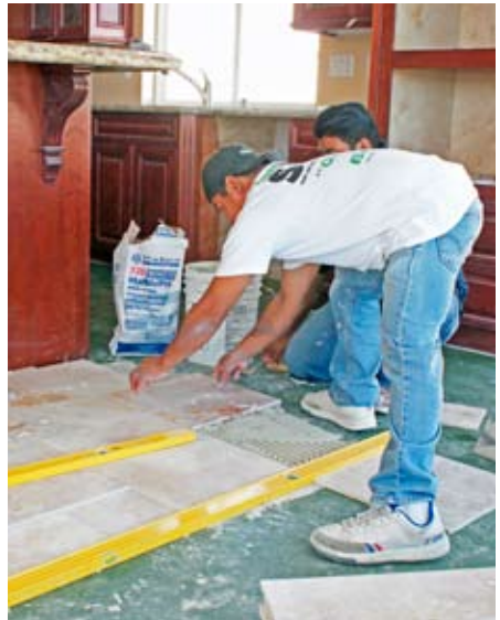
Tile is installed under the kitchen serving bar.
