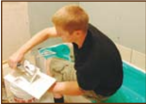
Buttering the tile with Mer-Krete's Mer-Stik adhesive.
