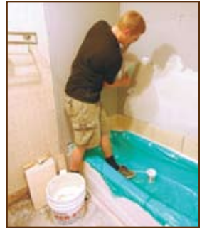
Applying Mer-Krete's Mer-Stik to shower stall area.
